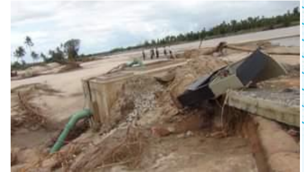
Damaged Borehole
