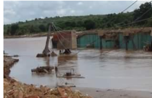
Downed Power Lines
