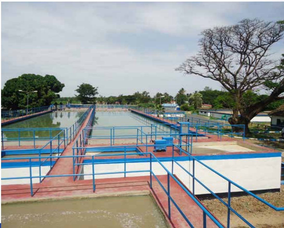
Dunga treatment plant: one of the projects in Kisumu
